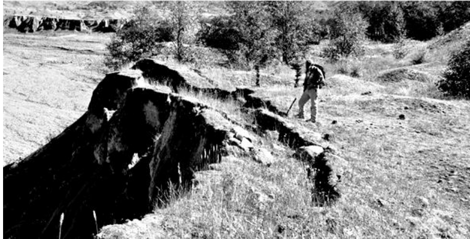
Klimets, Danny (2009) Tension Cracks . Photograph. https://search.creativecommons.org/photos/6902a3cb-cc5a-45ec-9b51-3a0b0b4457ed . Licensed under CC BY-NC-ND 2.0. https://creativecommons.org/licenses/by-nc-nd/2.0/?ref=ccsearch&atype=rich
